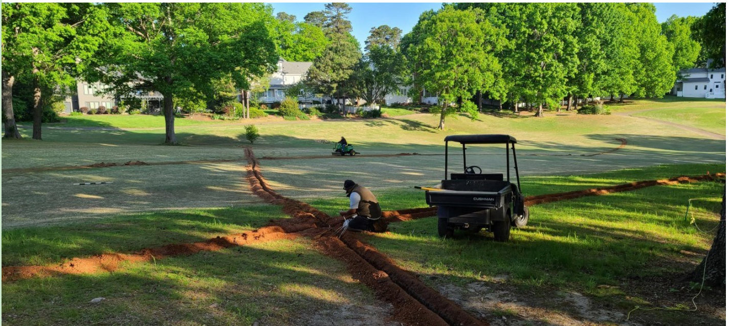
Laying irrigation wires on hole #14
